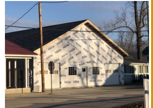
The SOS Mart will reopen this summer! Renovation is underway.
